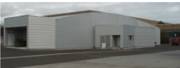
Fig 3. An External View of RMIT Industrial Wind Tunnel
