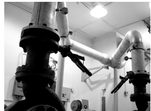
Fig 6: Modified Y-connection replacing T-connection
