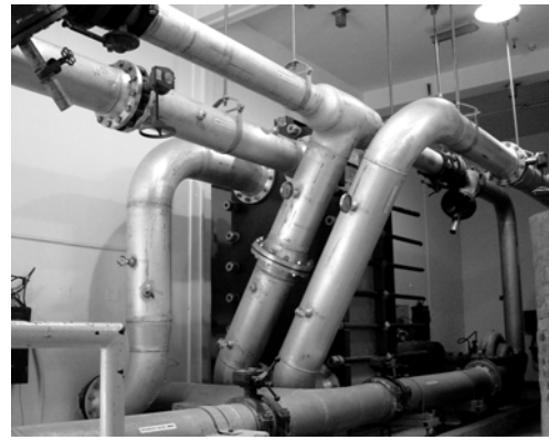
Fig 5: Plate type H/E with modified piping arrangements
