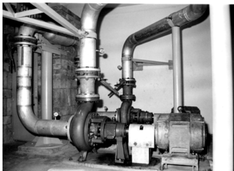
Fig 7: Modified pipe supports
