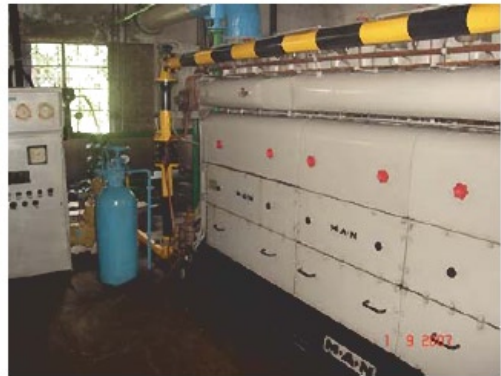
Dual Fuel Conversion of Diesel Generator
